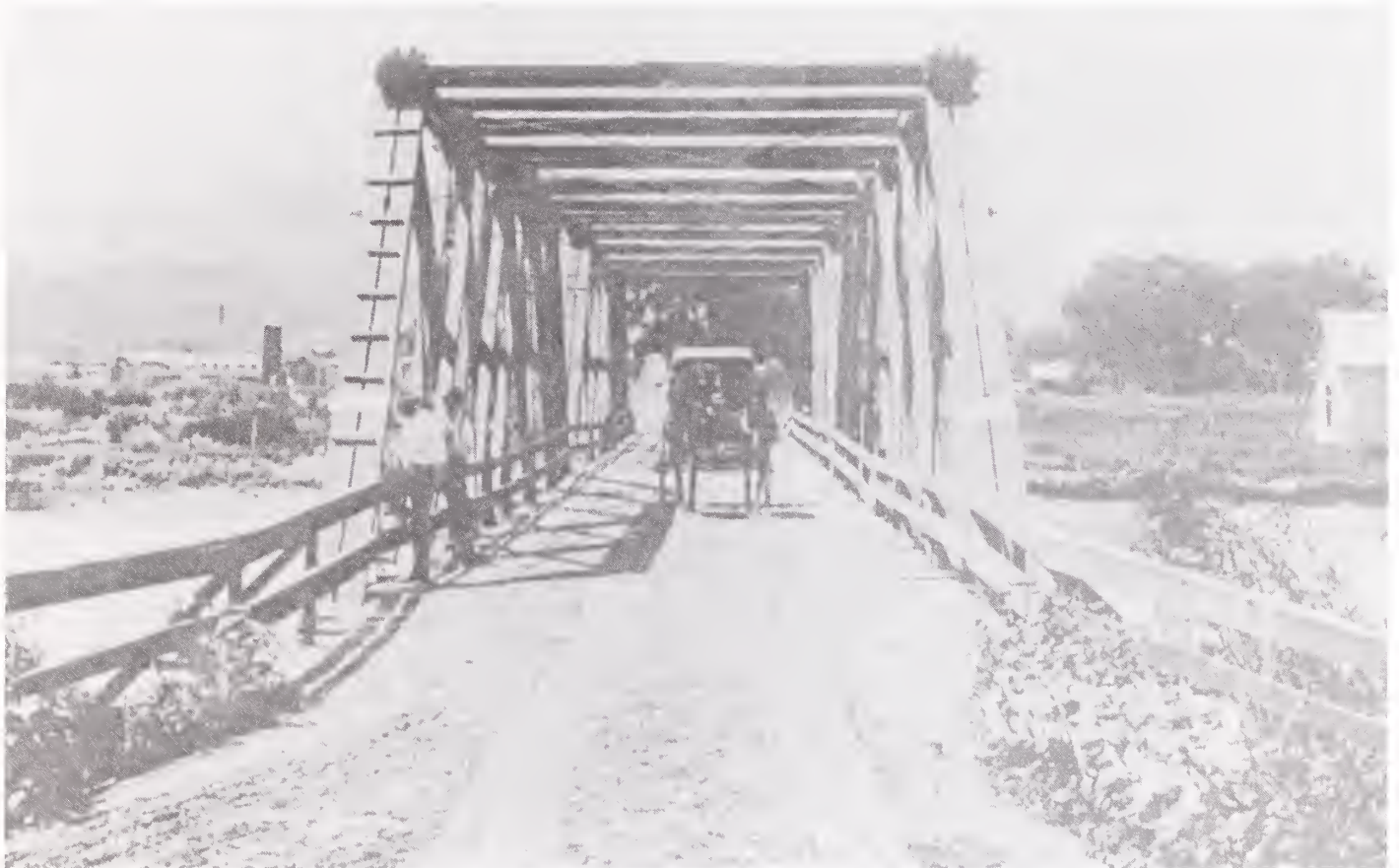
This wooden Howe truss bridge was located on the Clark's Fork of the Yellowstone River near Fromberg. Built in 1909, a reinforced concrete arch bridge replaced it in 1914 (Fromberg Service Club).
